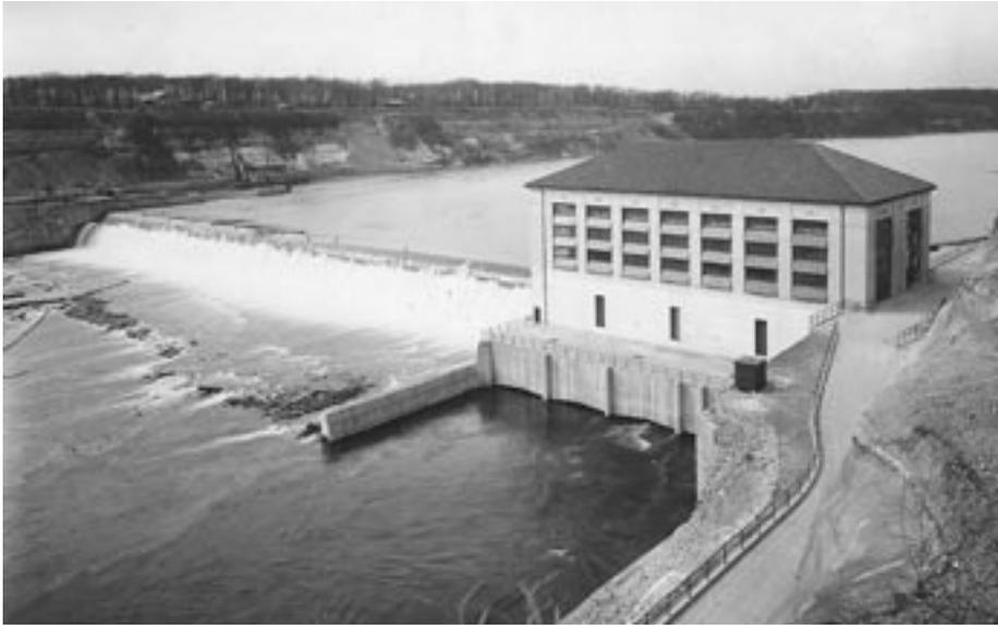
*After acquiring his industrial site and receiving the license to operate the hydroelectric plant, Ford rebuilt the foundation completed earlier by the Army Corps of Engineers. Photo courtesy of the author.*
