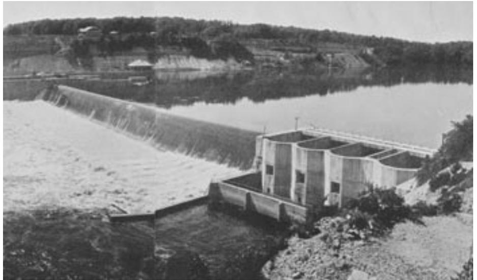
*View of Lock and Dam Number 1 showing the foundation for a hydroelectric plant completed six years before Ford purchased the adjoining site for his assembly plant. Image taken from the city of St. Paul's application to the Federal Power Commission in 1921, courtesy of the Minnesota Historical Society.*
